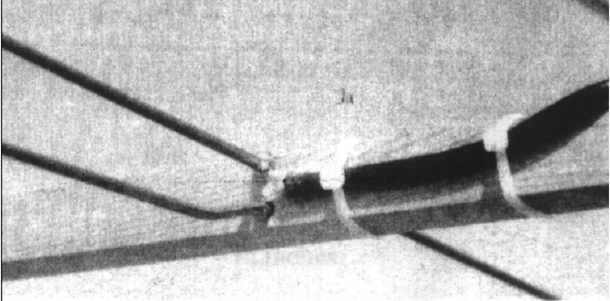
mounting of the feedline and driven element
